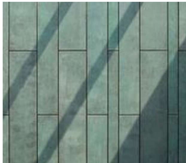
OXIDIZED COPPER CLADDING
