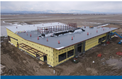
Exterior wall framing and sheathing
