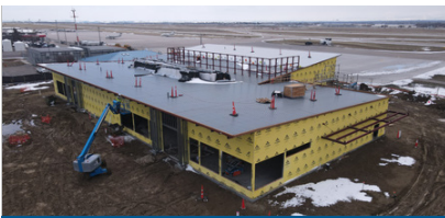
Terminal construction progress
