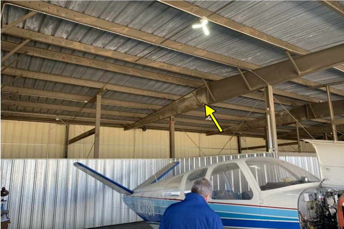
Figure 18 – IMG_6674 – Building 1, Unit 10 – Example wide-flange girder candidate for cleaning and inspection to evaluate extent of rust/deterioration damage.
