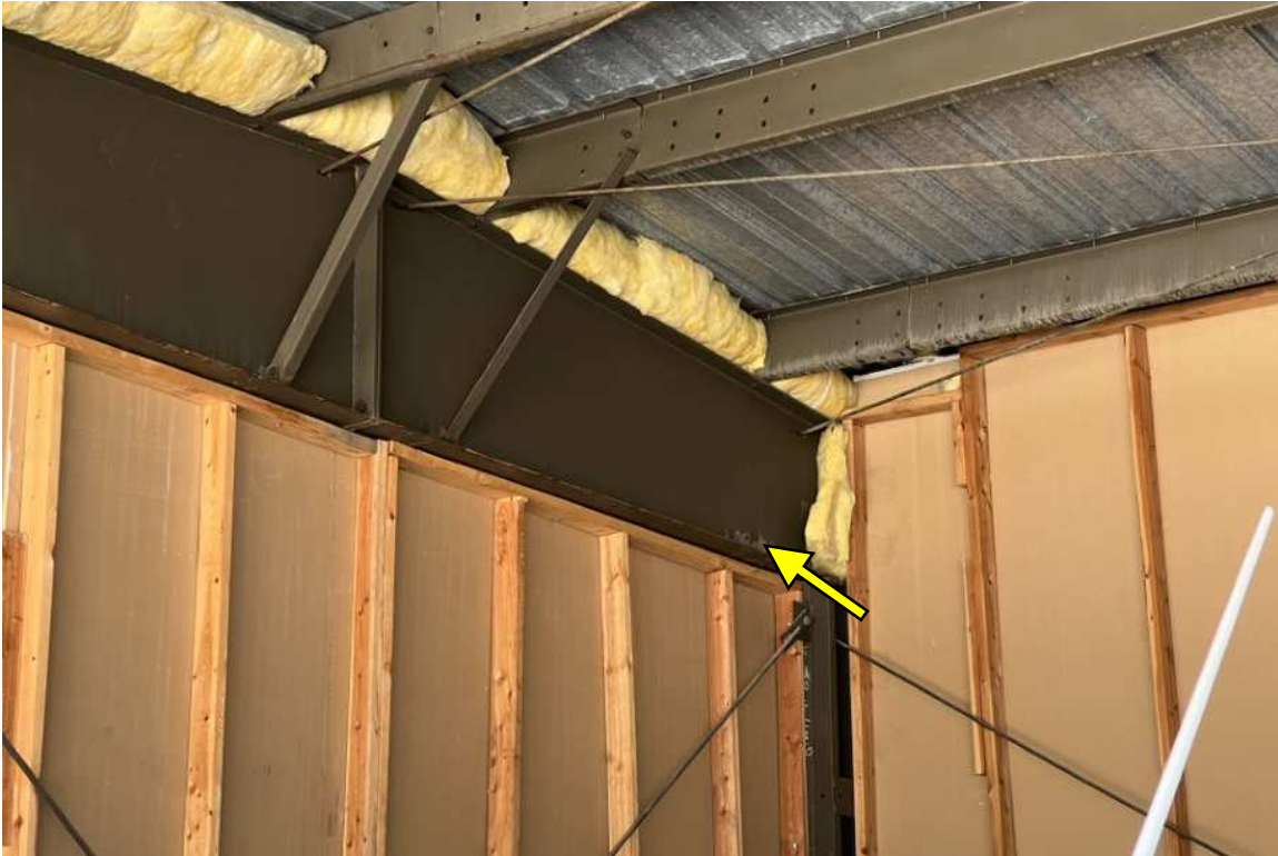
Figure 11 – IMG_5236 – Building 2, Unit 10 – Exemplar photograph of missing angle kicker bracing bottom flange of tapered wide-flange girder member.
