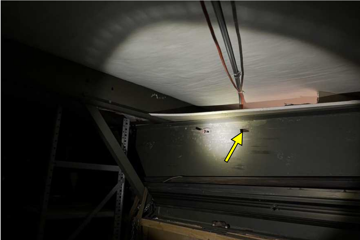
Figure 28 – IMG_5288 – Building 2, Storage unit adjacent to Unit 2 – Exemplar photograph of missing diaphragm bracing.
