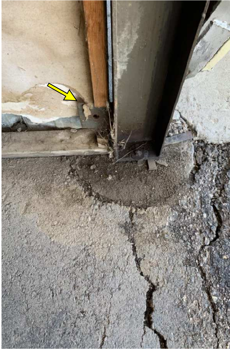
Figure 27 – IMG_6732 – Building 2, Unit 3 – Exemplar photograph of missing vertical tension rod element.
