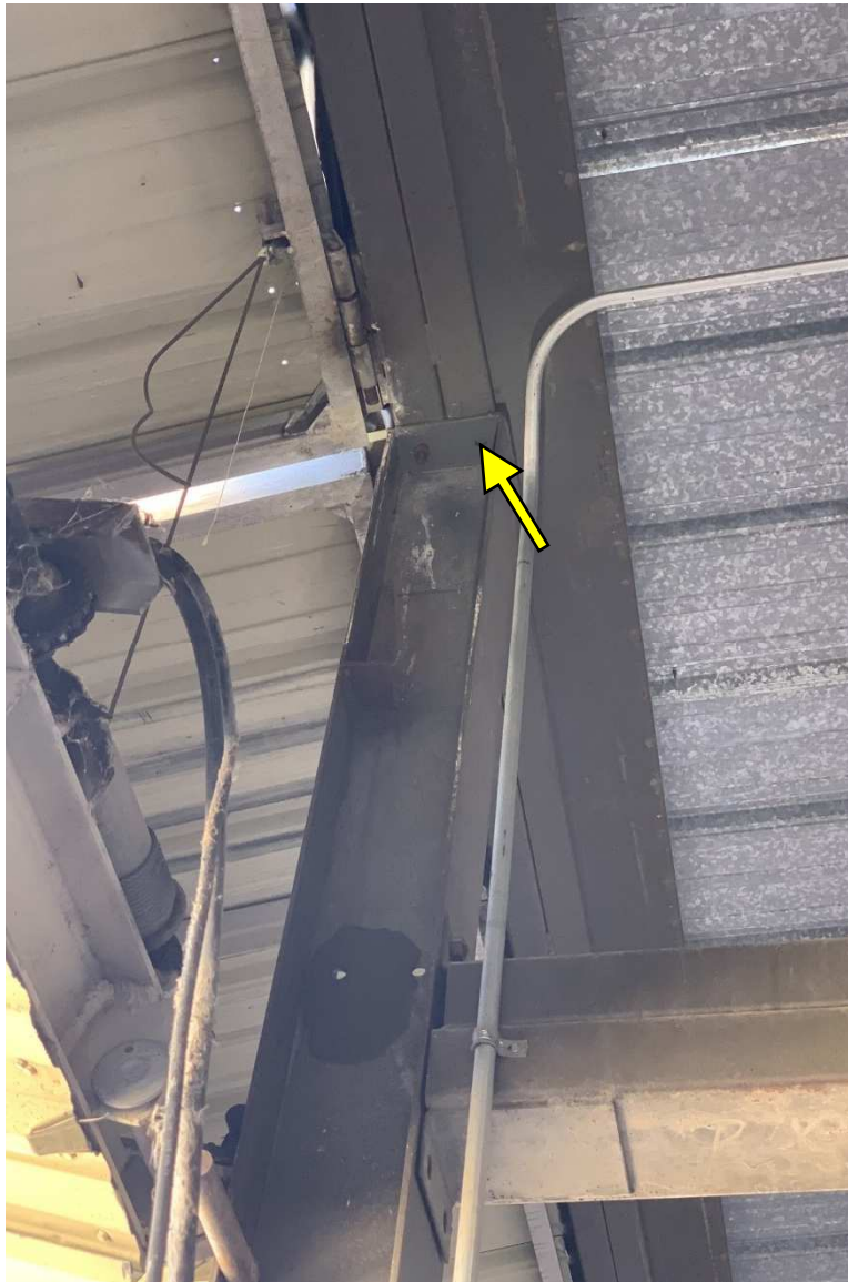
Figure 25 – IMG_6654 – Building 1, Unit 14 – Exemplar photograph of missing bolts in structural bolted connections.
