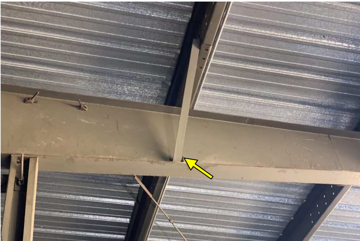
Figure 10 – IMG_6620 – Building 1, Unit 20 – Exemplar photograph of detached angle kicker bracing bottom flange of tapered wide-flange girder member.
