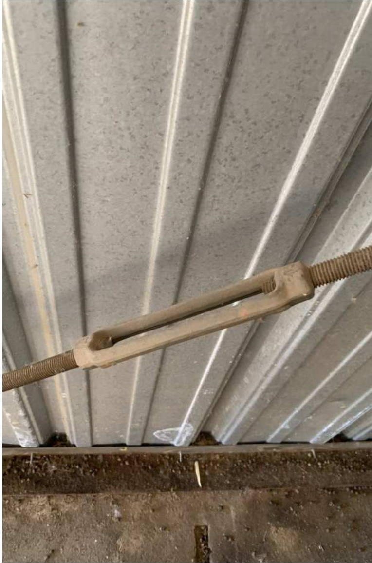
Figure 30 – IMG_6470 – Building 1, Storage unit adjacent to Unit 1 – Exemplar photograph of turnbuckle requiring snug hand tightening.
