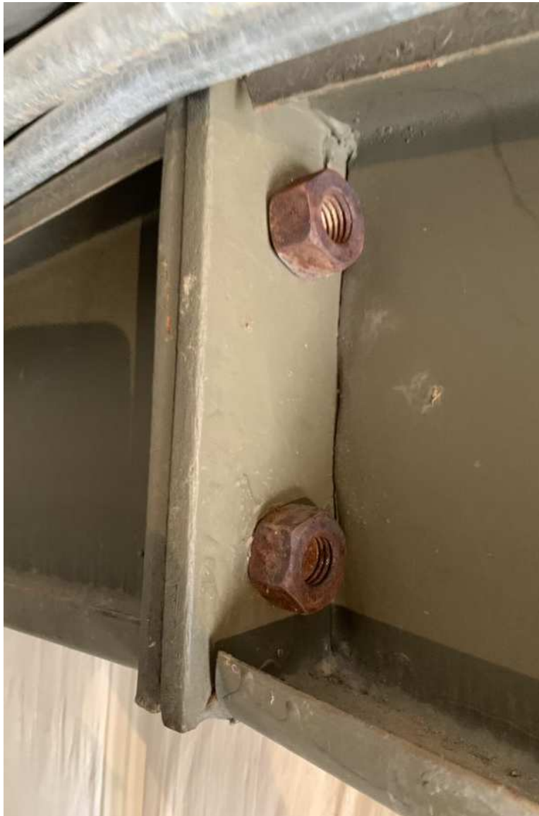
Figure 23 – IMG_6461 – Building 1, Storage unit adjacent to Unit 1 – Exemplar photograph of inadequate thread count above tightening nut.
