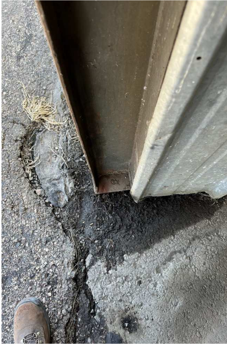
Figure 17 – IMG_5163 – Building 2, Unit 7 – Exemplar condition of detached anchorage (anchor connection failed due to corrosion; threads not protruding above nut due to column sitting on shims installed during, or post, construction; or both).
