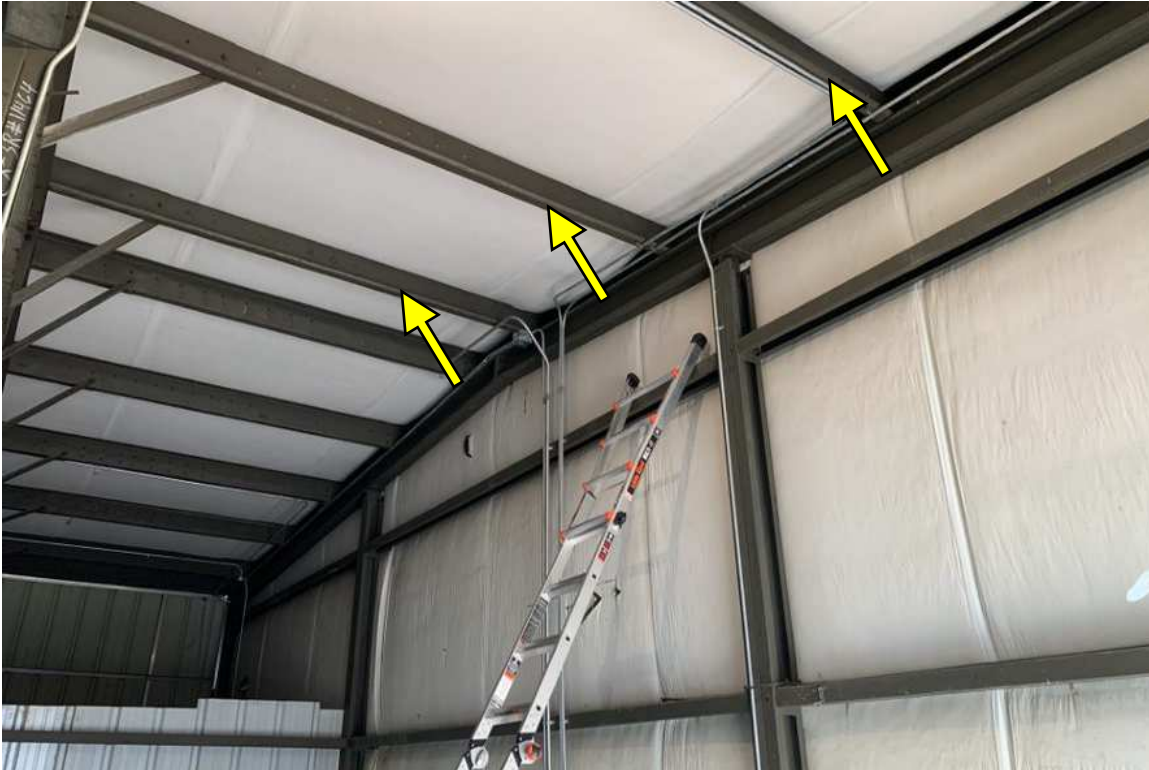
Figure 32 – IMG_6456 – Building 1, Storage adjacent to Unit 1 - Isolated roof framing members exhibiting deviations from the vertical ("rolling") -ongoing monitoring required.
