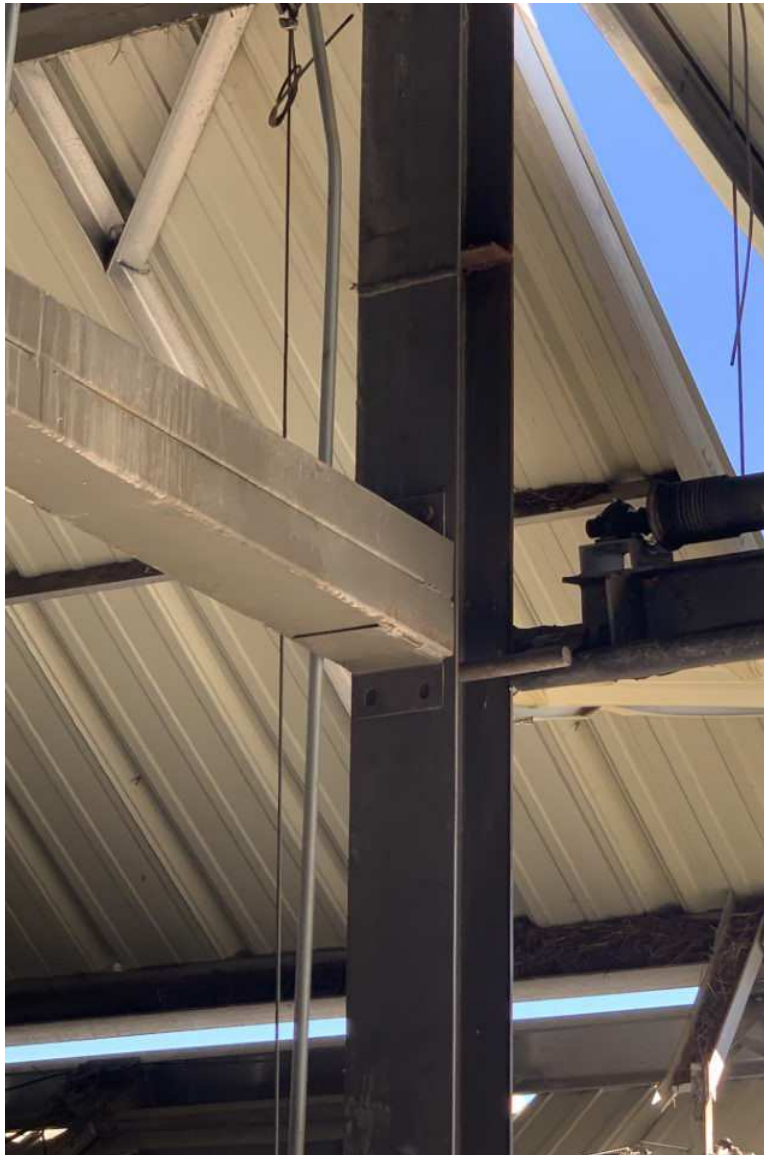
Figure 24 – IMG_6554 – Building 1, Unit 13 – Exemplar photograph of missing bolts in structural bolted connections.
