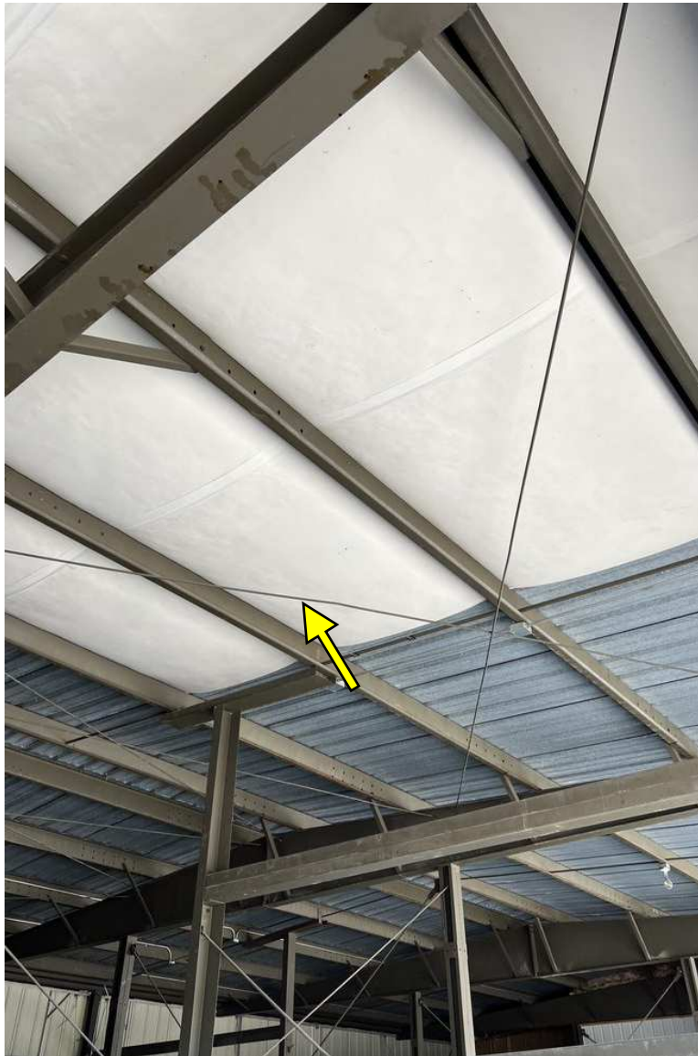
Figure 29 – IMG_5276 – Building 2, Unit 4 – Exemplar photograph of buckling of diaphragm bracing.
