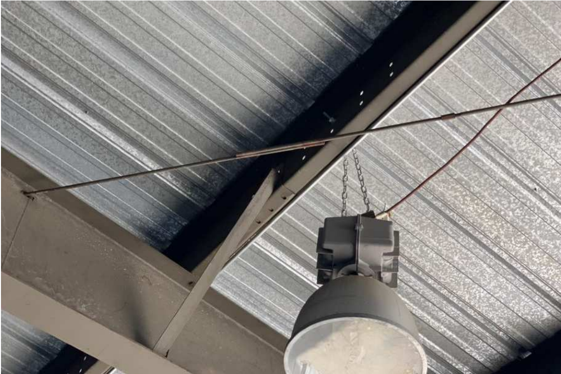
Figure 38 – IMG_6606 – Building 1, Unit 19 – Exemplar photograph of eccentric welded connection between two tension members in diaphragm bracing.
