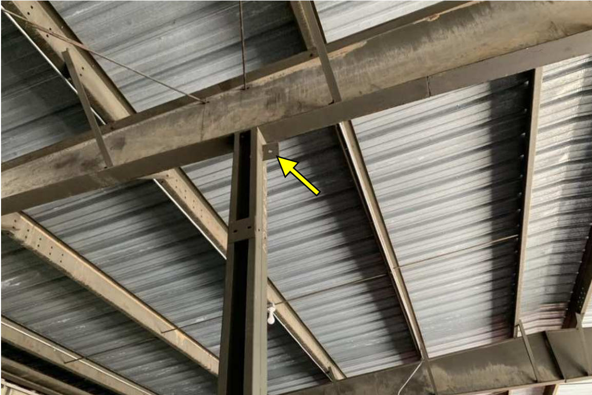
Figure 26 – IMG_6563 – Building 1, Unit 15 – Exemplar photograph of missing vertical tension rod element.
