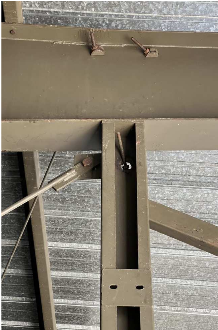
Figure 12 – IMG_5167 – Building 2, Storage unit adjacent to Unit 19 – Damaged lateral tension tie connection at column.
