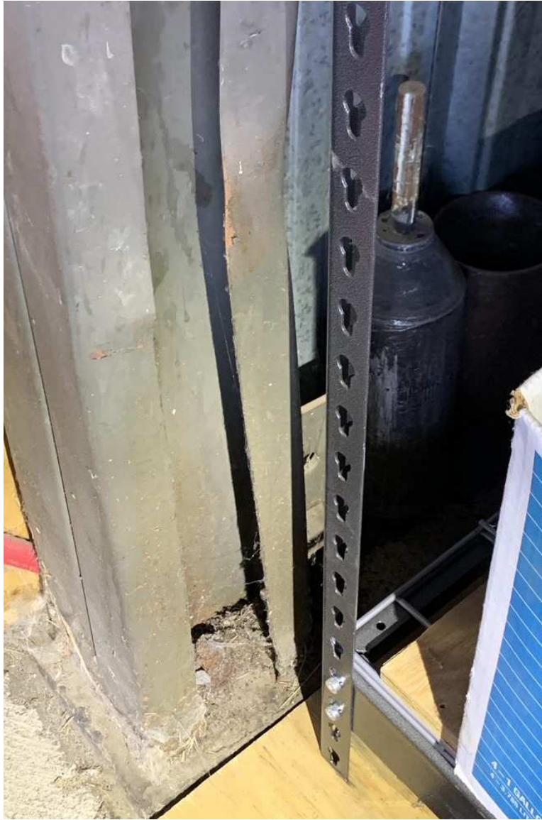
Figure 36 – IMG_6621 – Building 1, Unit 20 – Deformation, presumably due to impact, in structural member - ongoing monitoring required.
