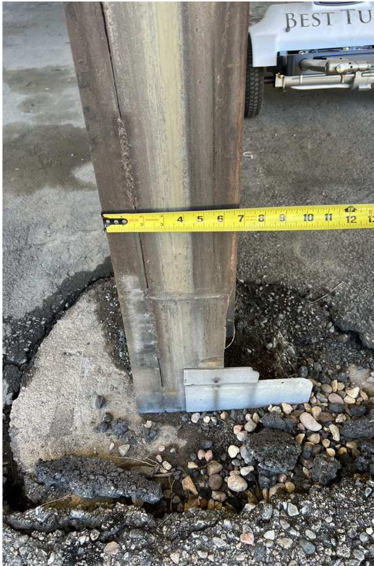
Figure 34 – IMG_5125 – Building 1, Unit 4 – Section loss in structural member - ongoing monitoring required.
