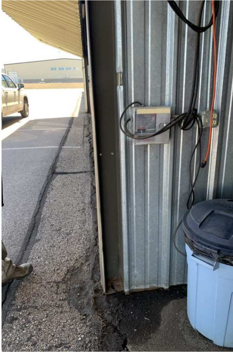
Figure 21 – IMG_6790 – Building 2, Unit 13 – Exemplar photograph of rotated column.
