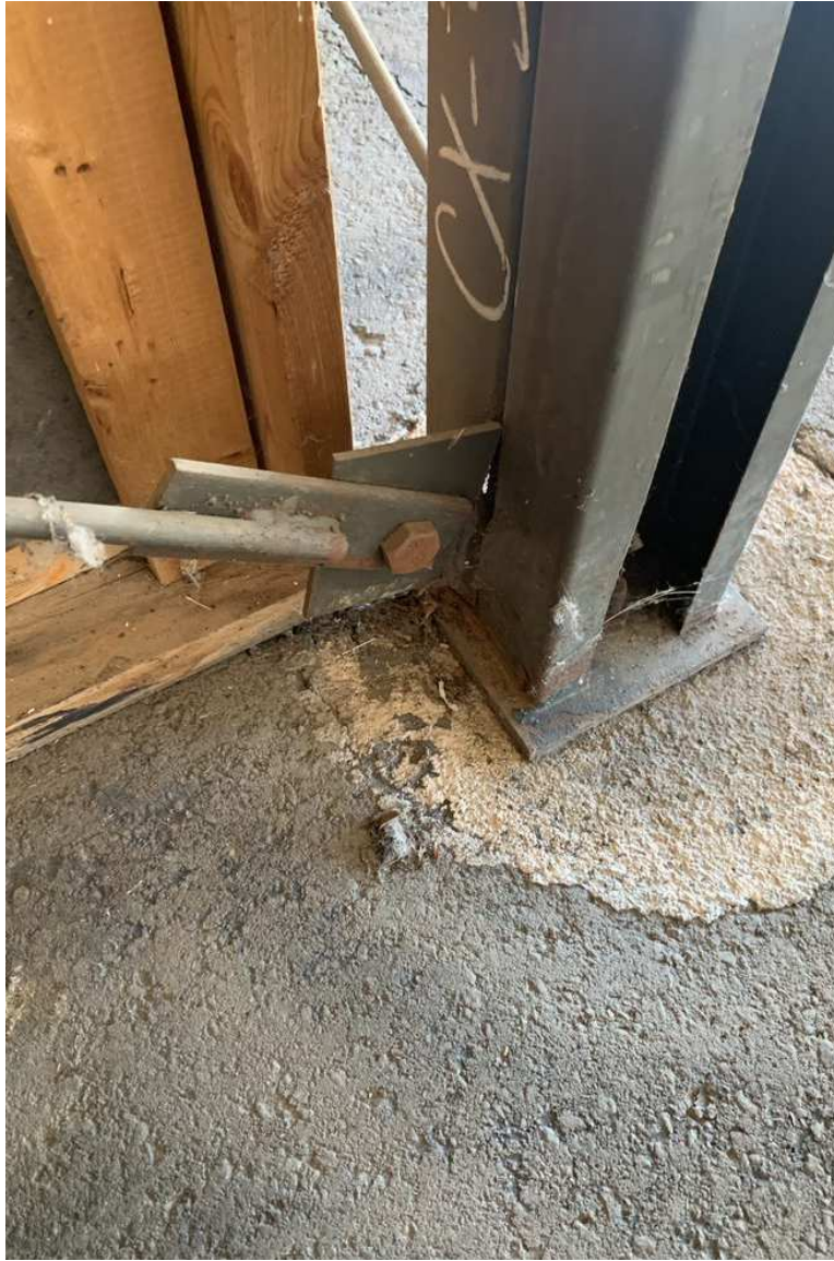
Figure 14 – IMG_6733 – Building 2, Unit 3 – Exemplar photograph of detached lateral brace plate connection to base of supporting column.
