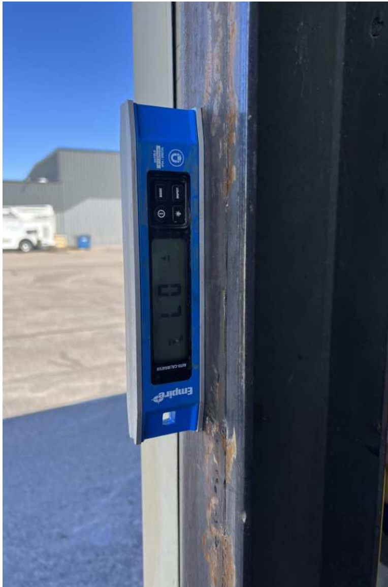
Figure 20 – IMG_5129 – Building 1, Unit 2 – Exemplar photograph of out-of-plumb column.
