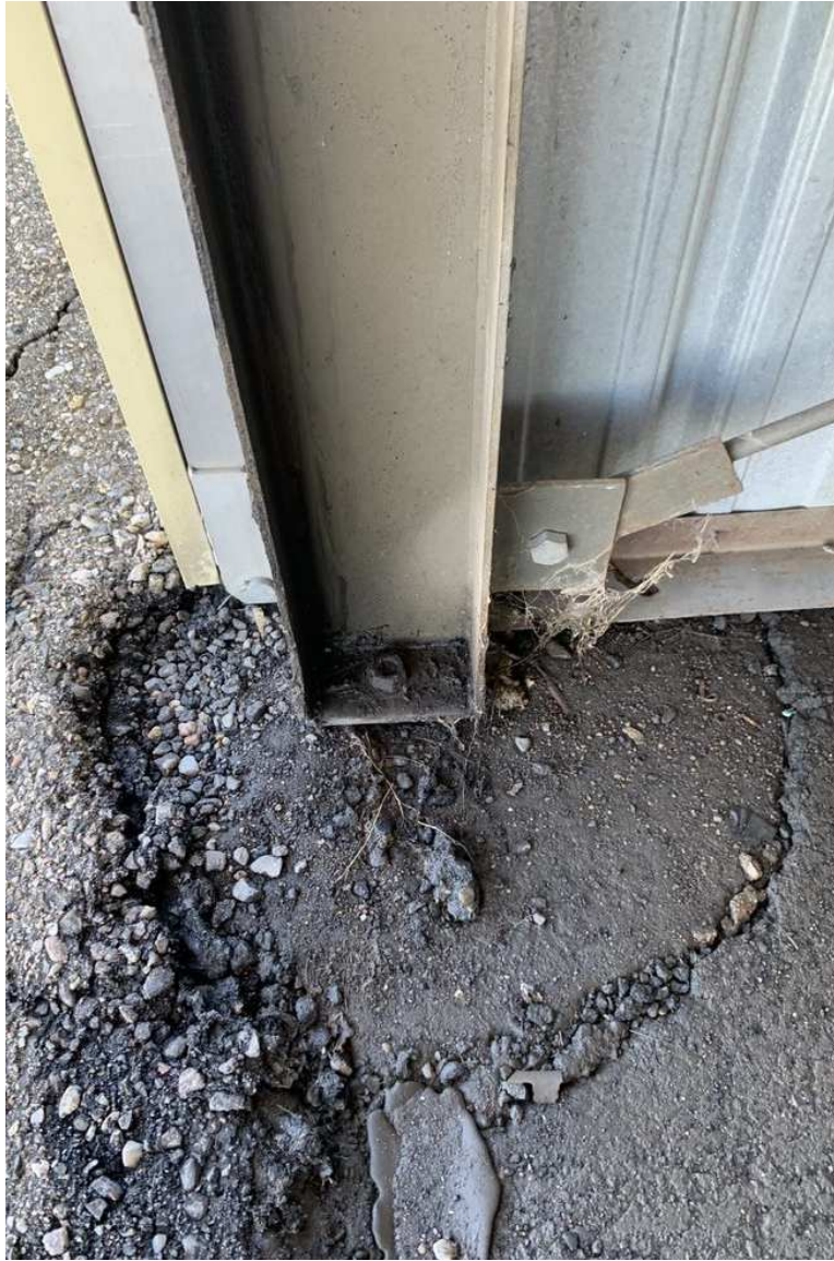
Figure 15 – IMG_6666 – Building 1, Unit 12 – Exemplar condition of damaged anchorage (threads not protruding above nut due to column sitting on shims installed during, or post, construction).
