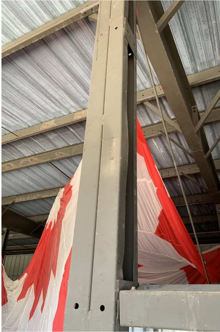
Figure 35 – IMG_6555 – Building 1, Unit 13 – Deformation, presumably due to impact, in structural member - ongoing monitoring required.
