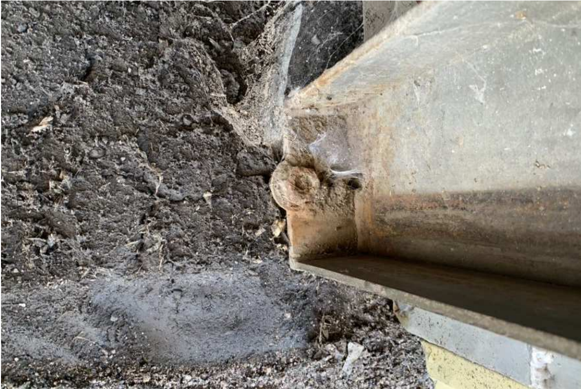
Figure 16 – IMG_6751 – Building 2, Unit 7 – Exemplar condition of detached anchorage (anchor bolt originally placed too near edge of plate and subject to corrosion).
