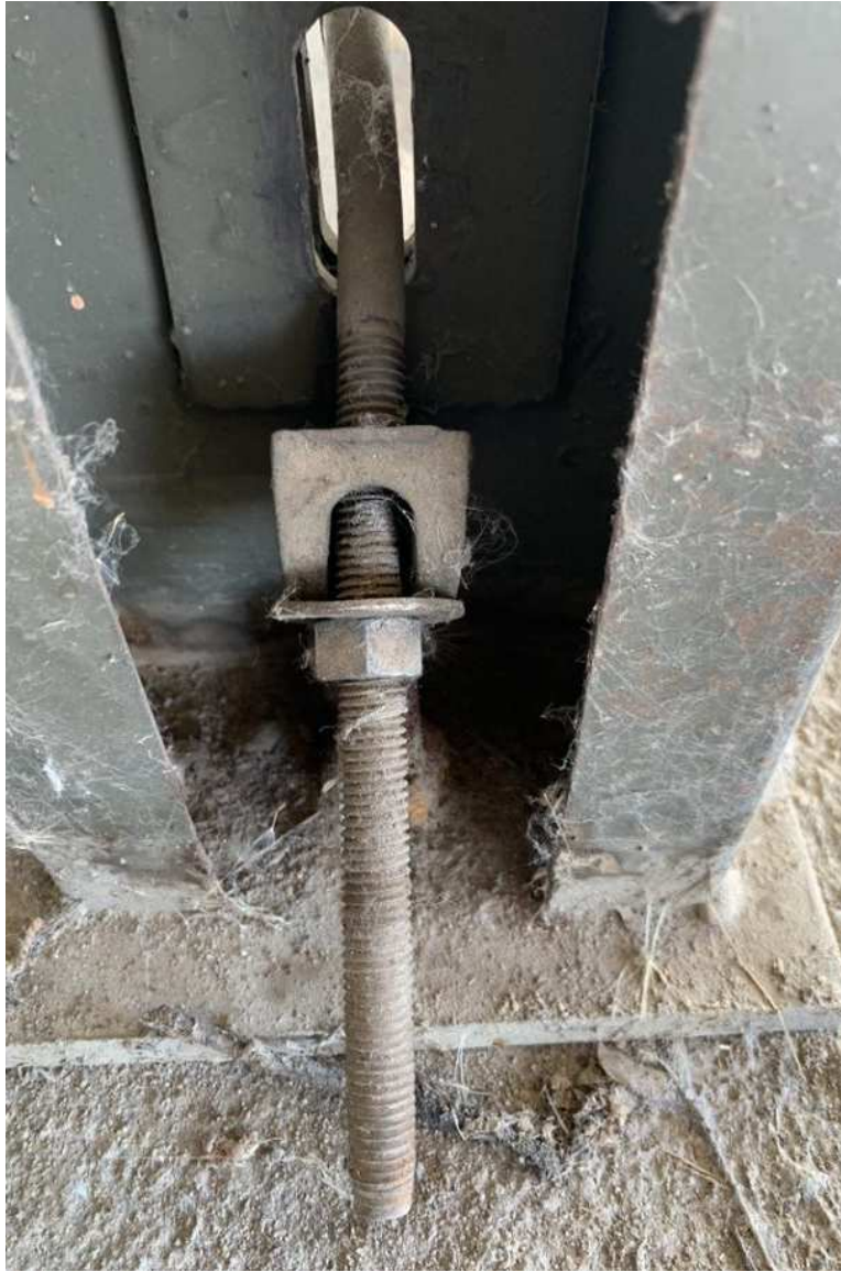
Figure 31 – IMG_6481 – Building 1, Storage unit adjacent to Unit 1 – Exemplar photograph of tension rod column connection requiring tightening.
