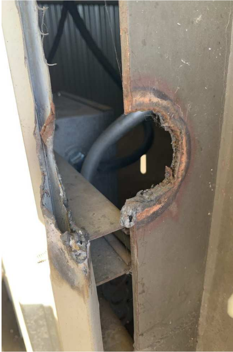
Figure 33 – IMG_6492 – Building 1, Unit 3 – Section loss in structural member - ongoing monitoring required.
