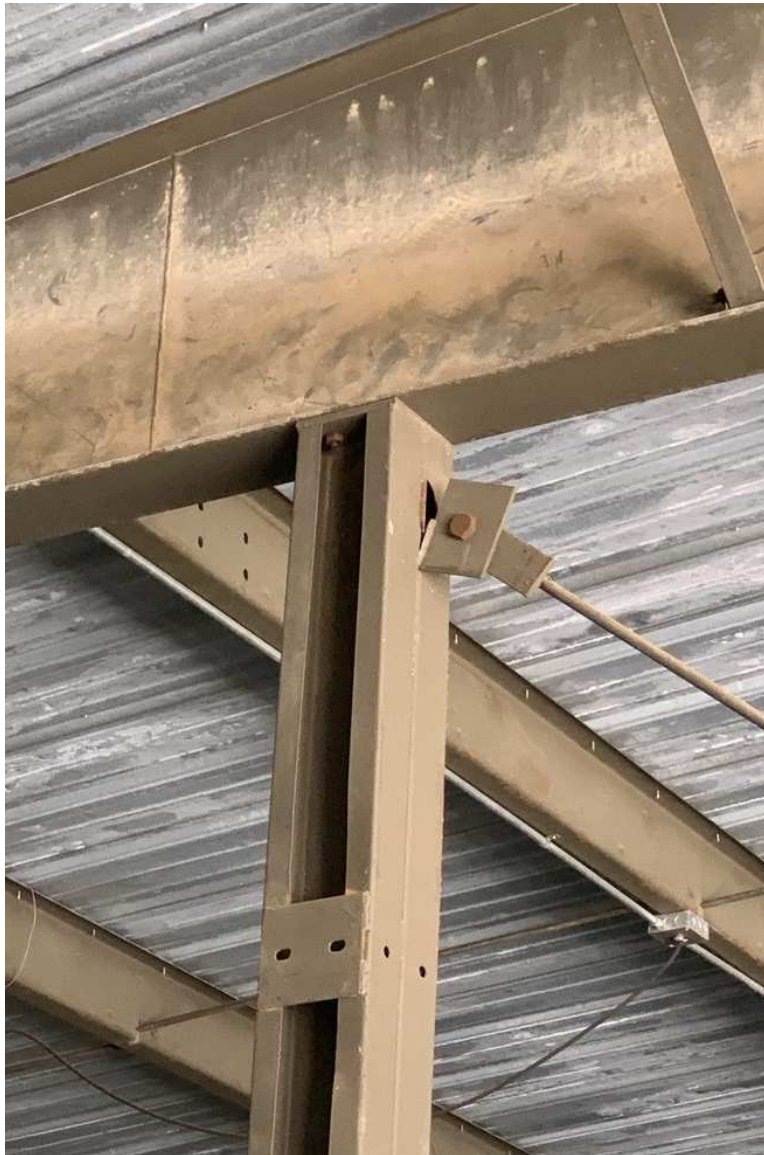
Figure 13 – IMG_6513 – Building 1, Unit 7 – Exemplar photograph of detached lateral brace plate connection to top of supporting column.
