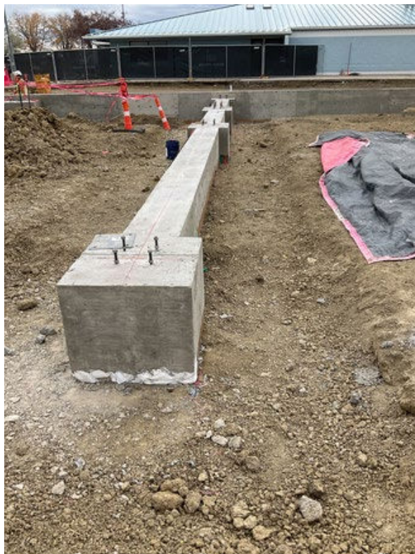
10/12/2023 Form work removal (Grade Beam 3)
