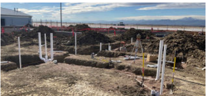
Underslab sanitary drain installation
