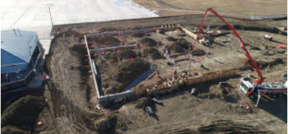
Building foundation progress
