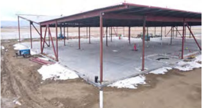
Steel framing erection
