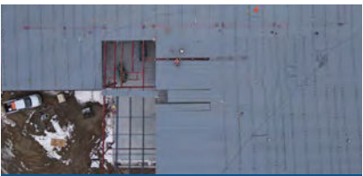
Roof decking installation
