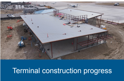
Completed roof decking
